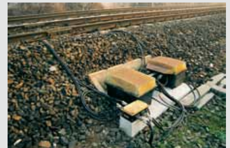
Electrical connection of underground metal structures to rails
