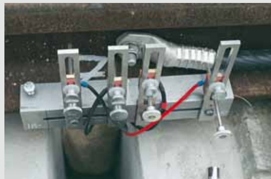
On site Testing
